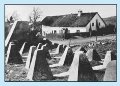
▲ The large concrete blocks with teeth were part of a road block formed by inserting steel girders into the gaps between the teeth. The barrier blocked the road leading from Großkampenberg to the present starting point of the Siegfried Line hiking trail and was located directly at the junction of the road from Kesfeld. Today you can still see the house in the background on the other side of the road.
