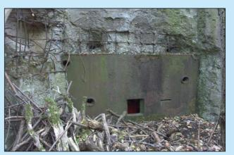
▲ Three shots from a 76 mm cannon smoothly penetrated the embrasure plate of soft rolled steel
