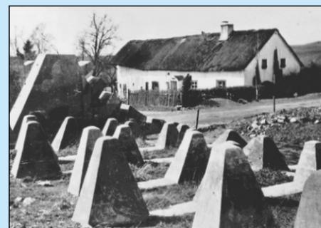
▲ *The large concrete blocks with teeth were part of a road block formed by inserting steel girders into the gaps between the teeth. The barrier blocked the road leading from Großkampfenberg to the present starting point of the Siegfried Line hiking trail and was located directly at the junction of the road from Kesfeld. Today you can still see the house in the background on the other side of the road.*
