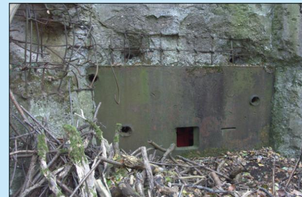
▲ Three shots from a 76 mm cannon smoothly penetrated the embrasure plate of soft rolled steel.
